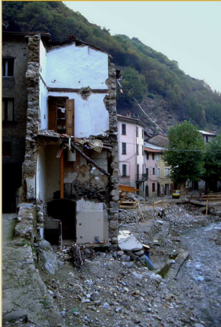
38 - Fornovolasco: case distrutte lungo la Tùrrite destroyed houses along the Tùrrite river
