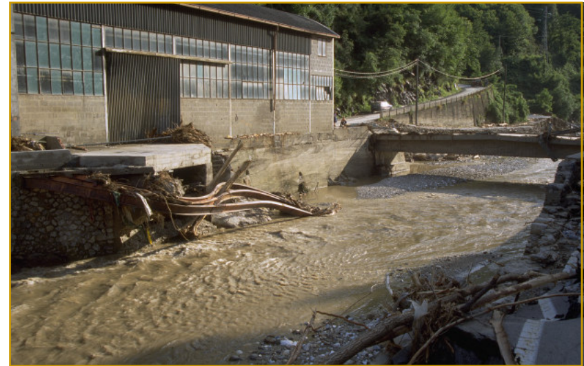
47 - Valentosa: ponte distrutto e ferro piegato dalla piena bridge destroyed and iron bent by the river overflow
